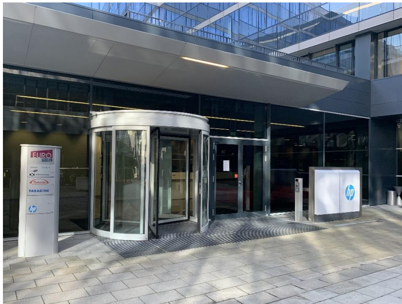
Picture 2 Entrance Paradine GmbH
